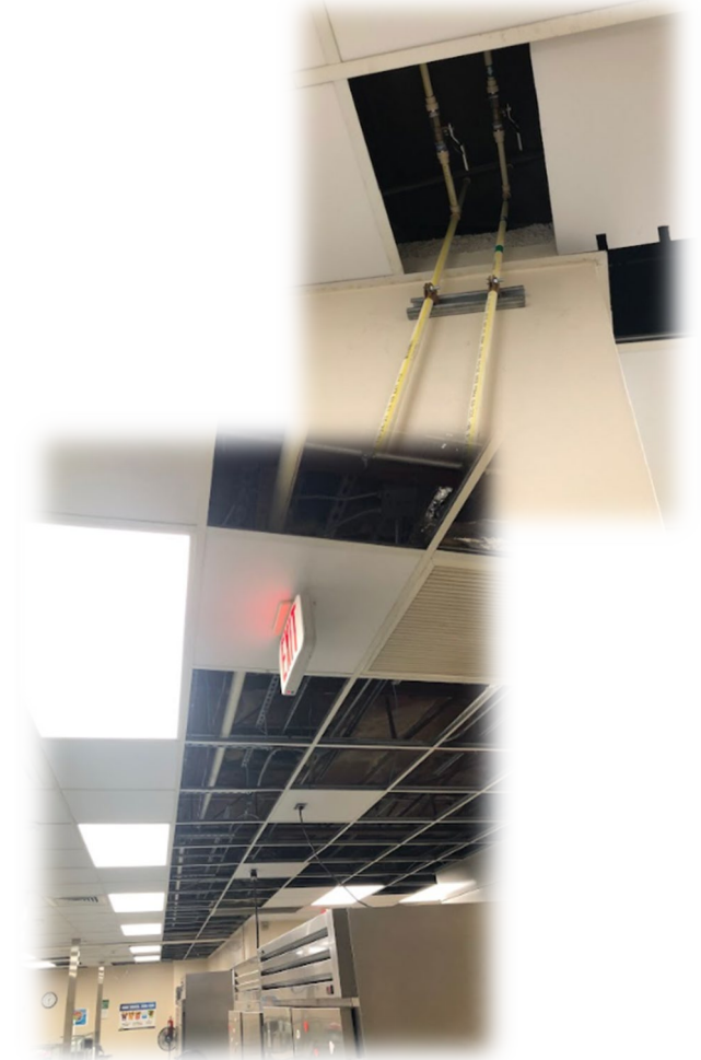
Fort Myers Middle Plumbing Renovation
